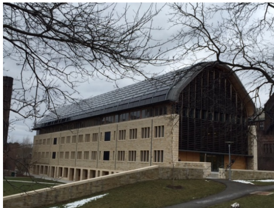
Solar roof, Yale University
